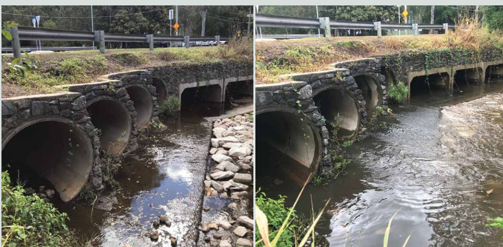
Figure 2. Depth and velocity are highly dynamic in the field. These images are of the same culvert taken less than 24 hours apart, and show how the depth and velocity changes over time, but also that it can differ between cells within the same culvert. Images: Jabin Watson
